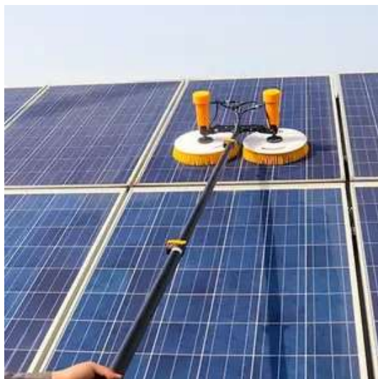
Fig.1. Special hand brush for cleaning the surface of solar panels.
